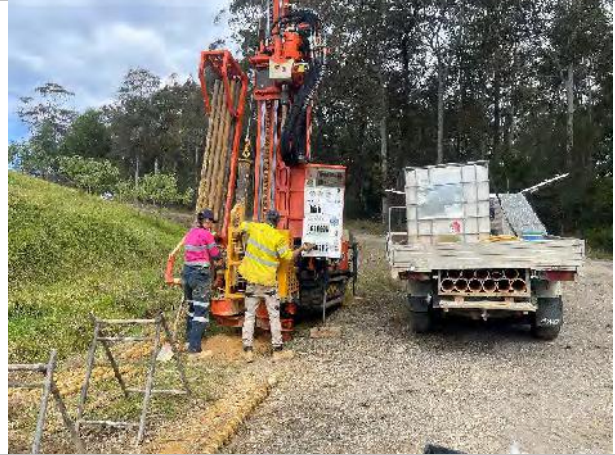
Photo 6: Drilling rig setup at BH10.
