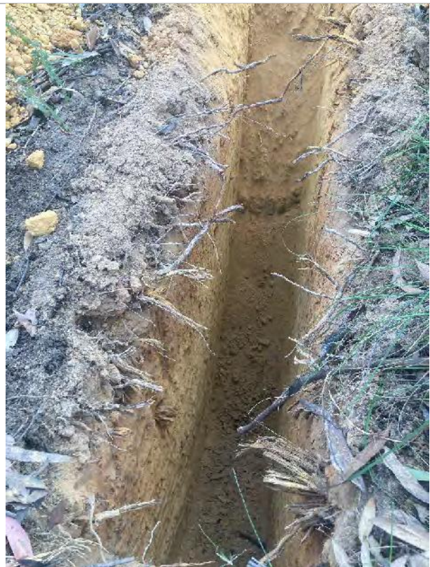
Photo 8: Test pit TP02 following excavation.
